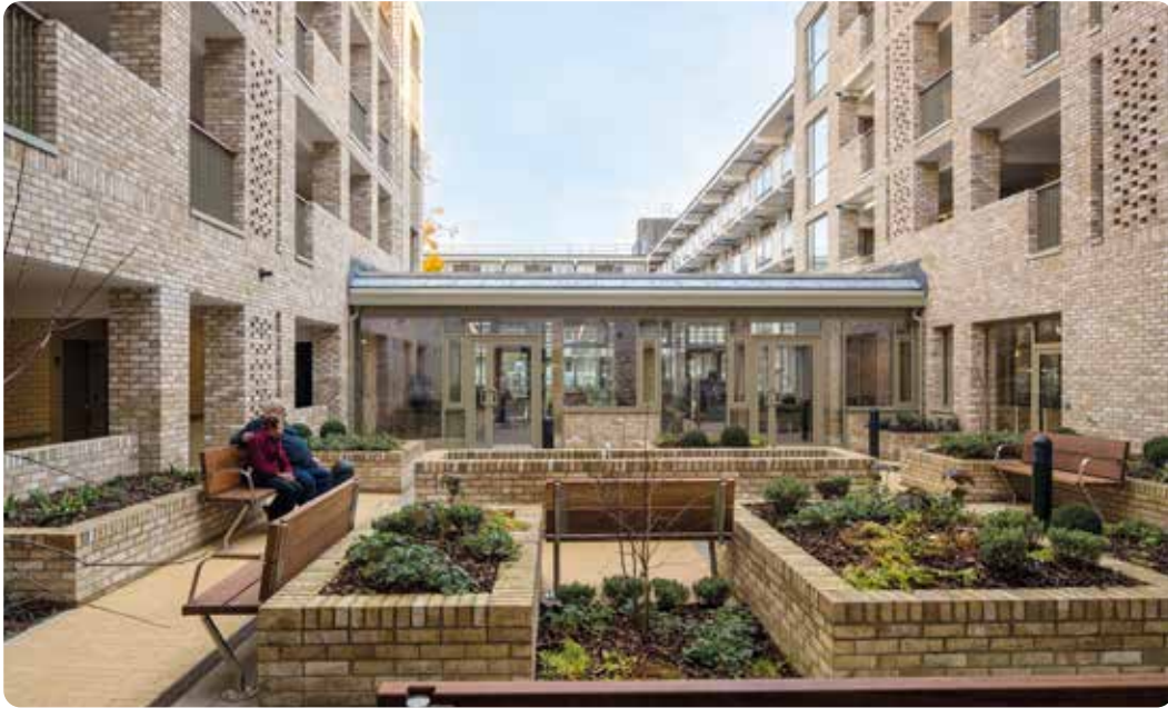
Courtyard garden in extra care scheme connected to the resident dining area
