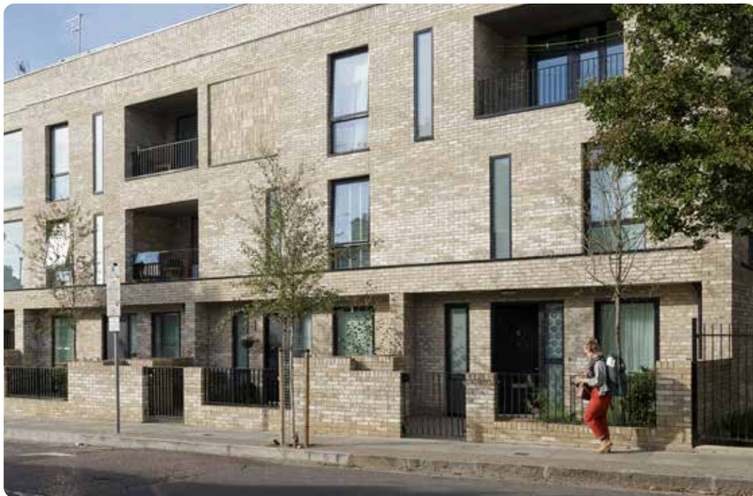
Duplex homes at ground floor with dedicated area for bin storage within front garden
