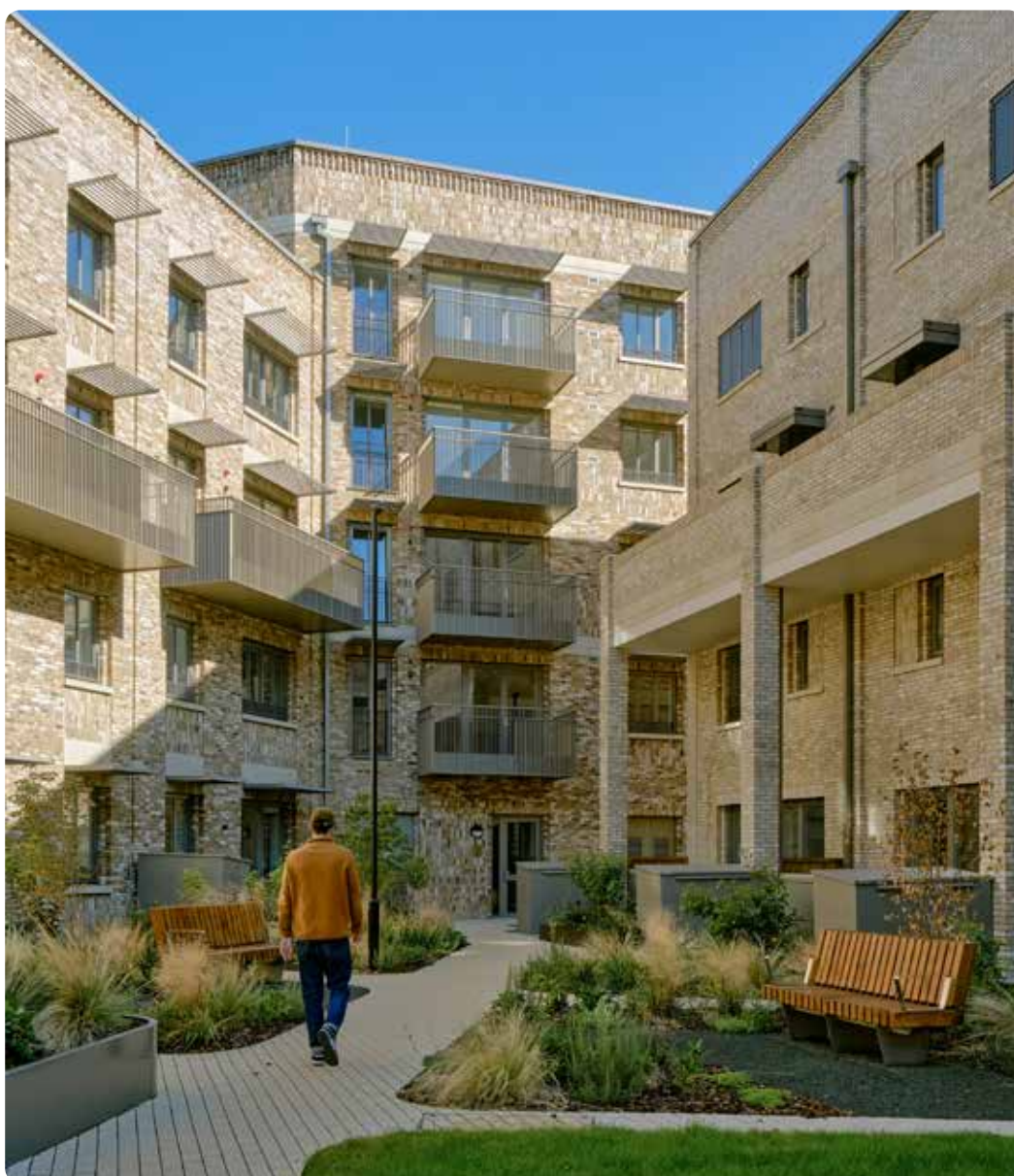
Window proportions and details relate to orientation, smaller windows face north and larger windows face south and west, incorporating shading
