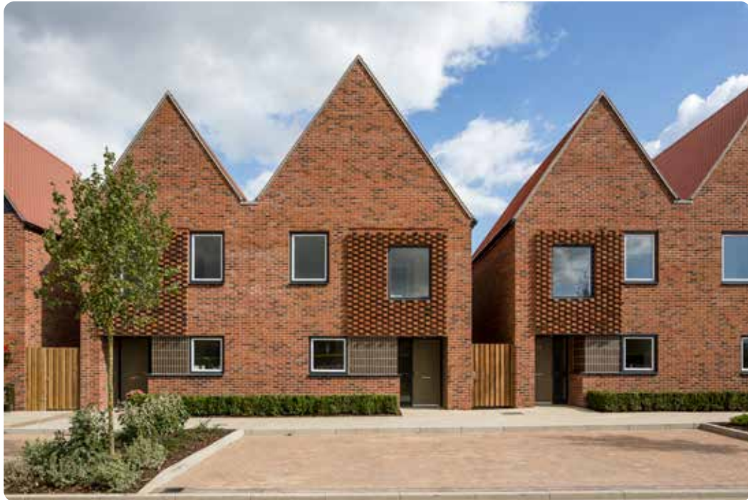
Houses using durable materials, with concealed meter cupboards and rainwater pipes
