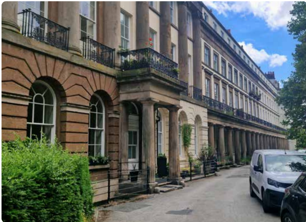
Retained, historic porticoes in Gambia Terrace
