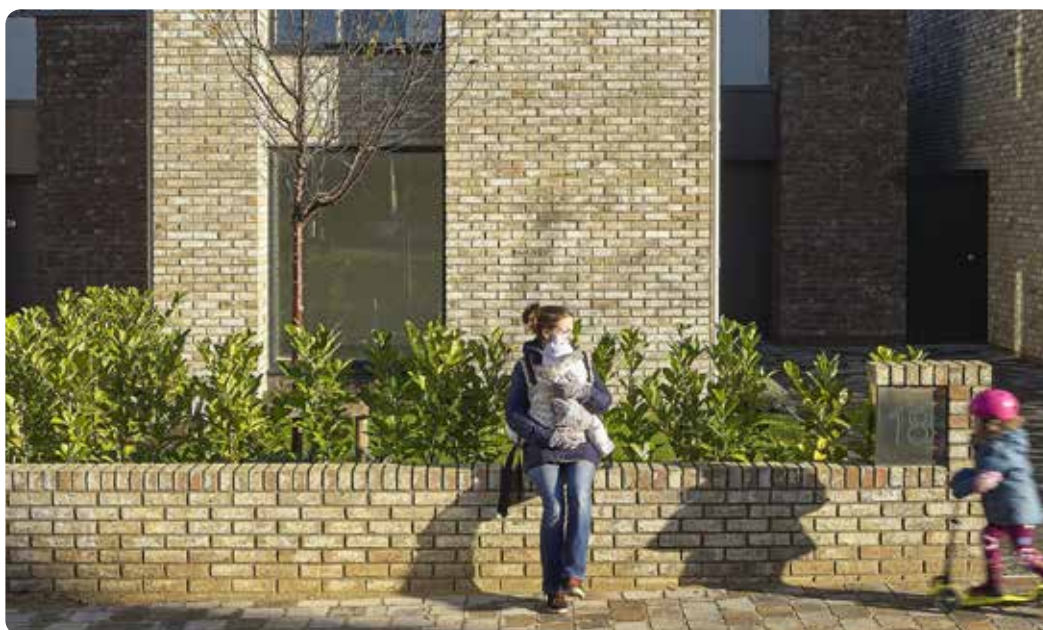
Front boundary of brick with evergreen hedge and integrated signage
