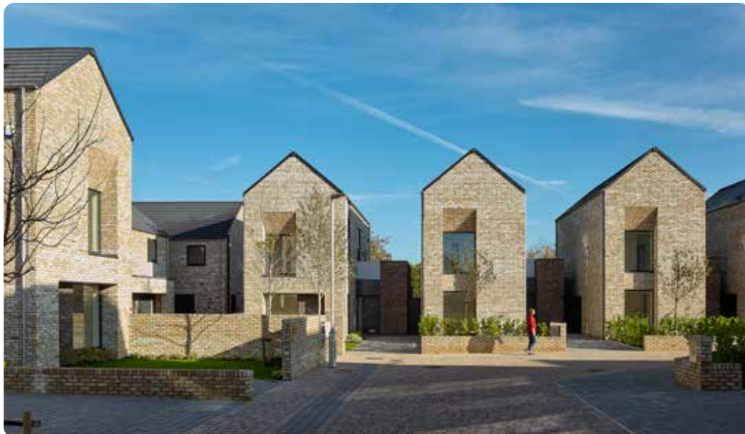
Shallow plots with innovate housing layouts enable a higher-density on this small infill site
