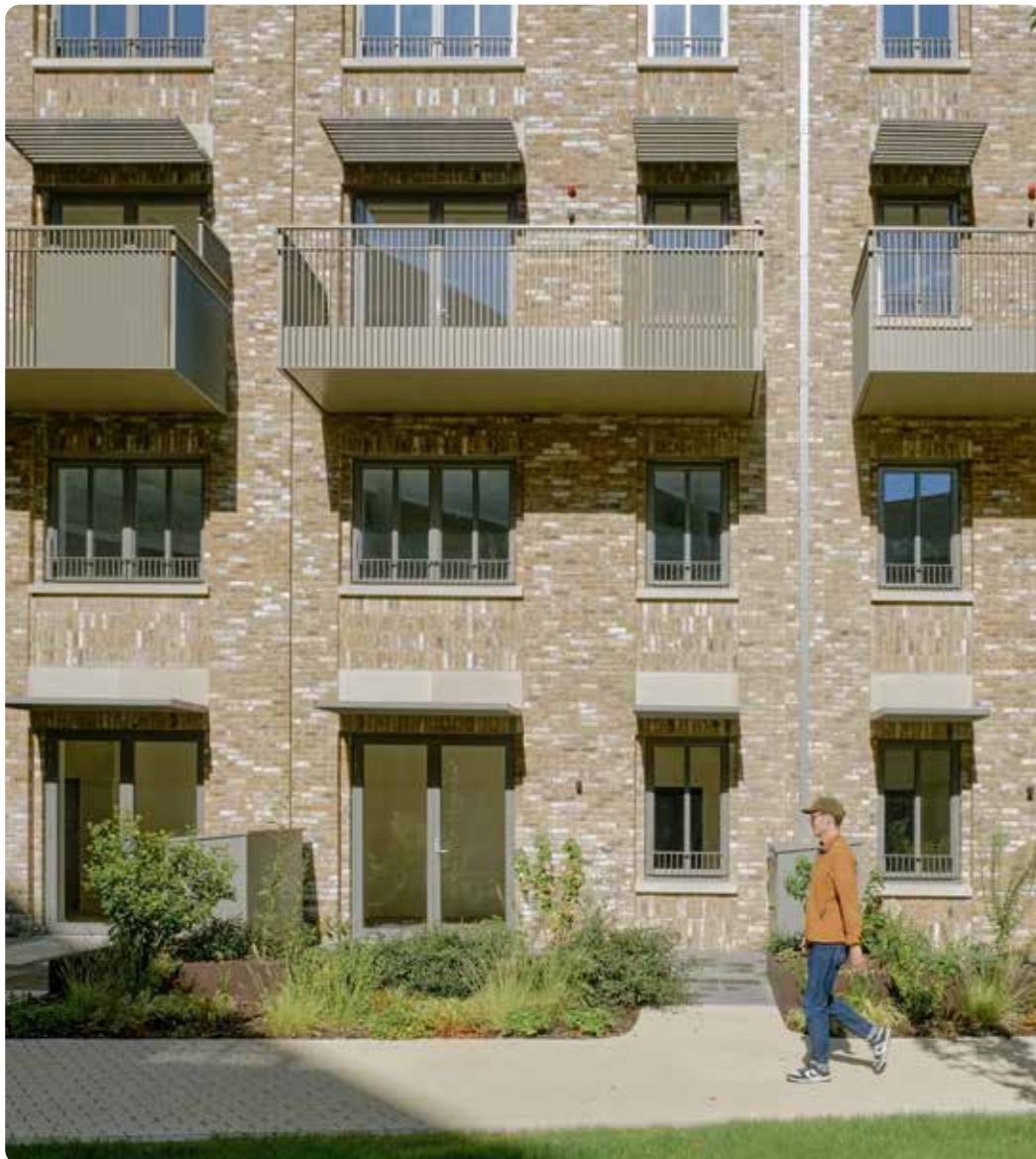
Balconies and fixed louvers on south facing windows provide shade for south facing windows
