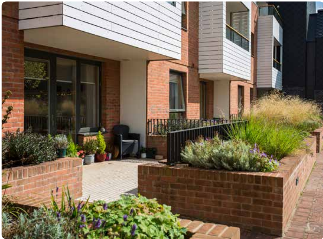
Independent living scheme where first floor balconies provide shelter and shade to the private amenity for homes below and private gardens have direct access to communal garden
