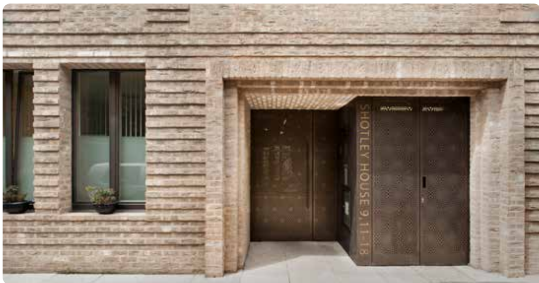
Doors to refuse store are easily accessible from core entrance but set back and set away from habitable rooms
