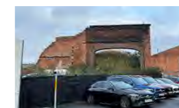
Fig 13 Warehouse walls retained as part of the new Canal Square
