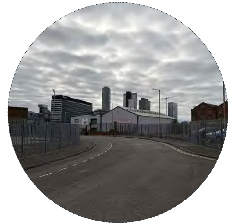
Fig 104 Pumpfields Road today
