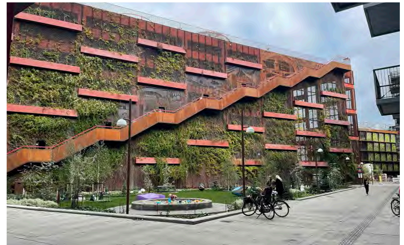
Fig 130 Mobility Hub designed to be fully integrated within its residential surroundings with green façades and a public playground at rooftop level.
