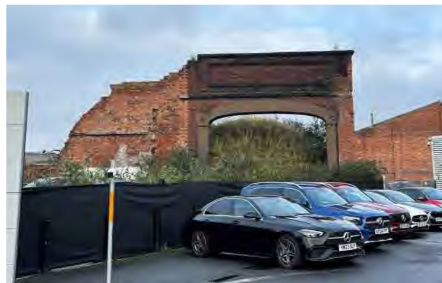
Fig 13 Warehouse walls retained as part of the new Canal Square
