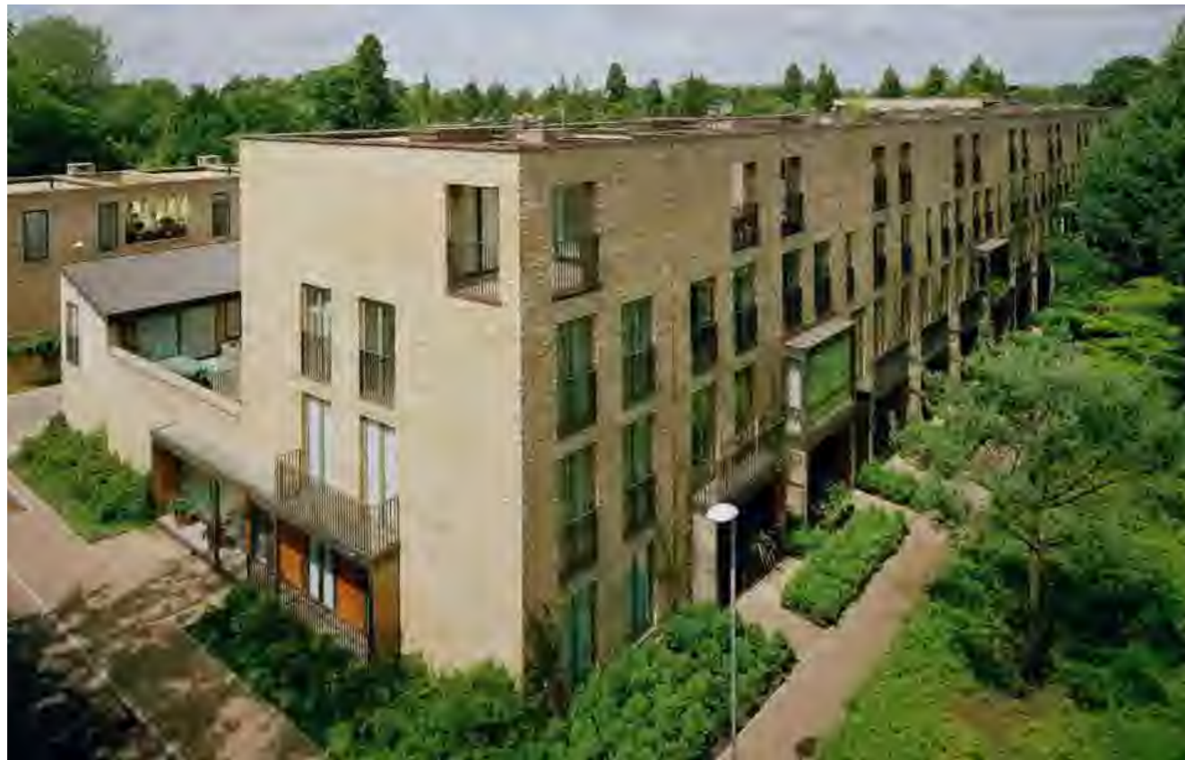
Fig 97 Four storey building along a linear park with planting defining front gardens
