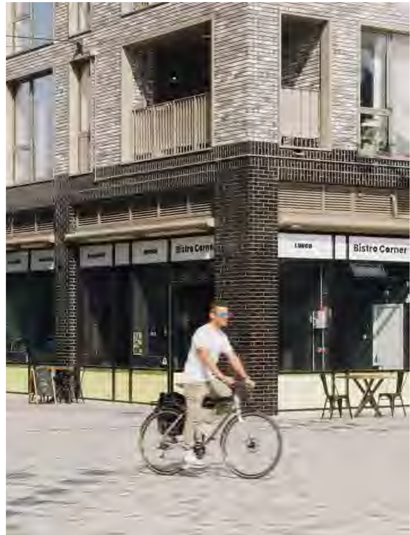
Fig 127 The ground floor's non-residential use is expressed through a change in brick colour, creating visual distinction
