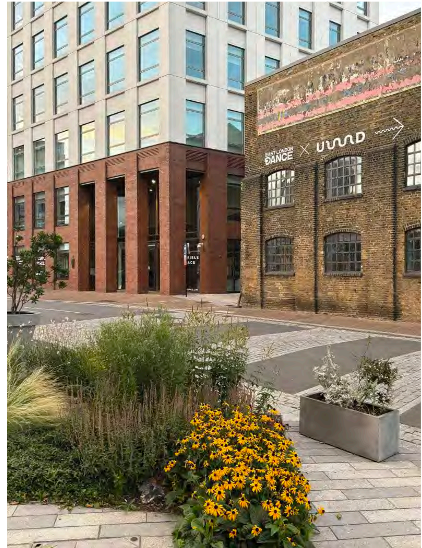
Fig 118 The façade design of the new mixed-use building takes cues from the adjacent retained warehouse, incorporating a two-storey base with a rhythm defined by piers.
