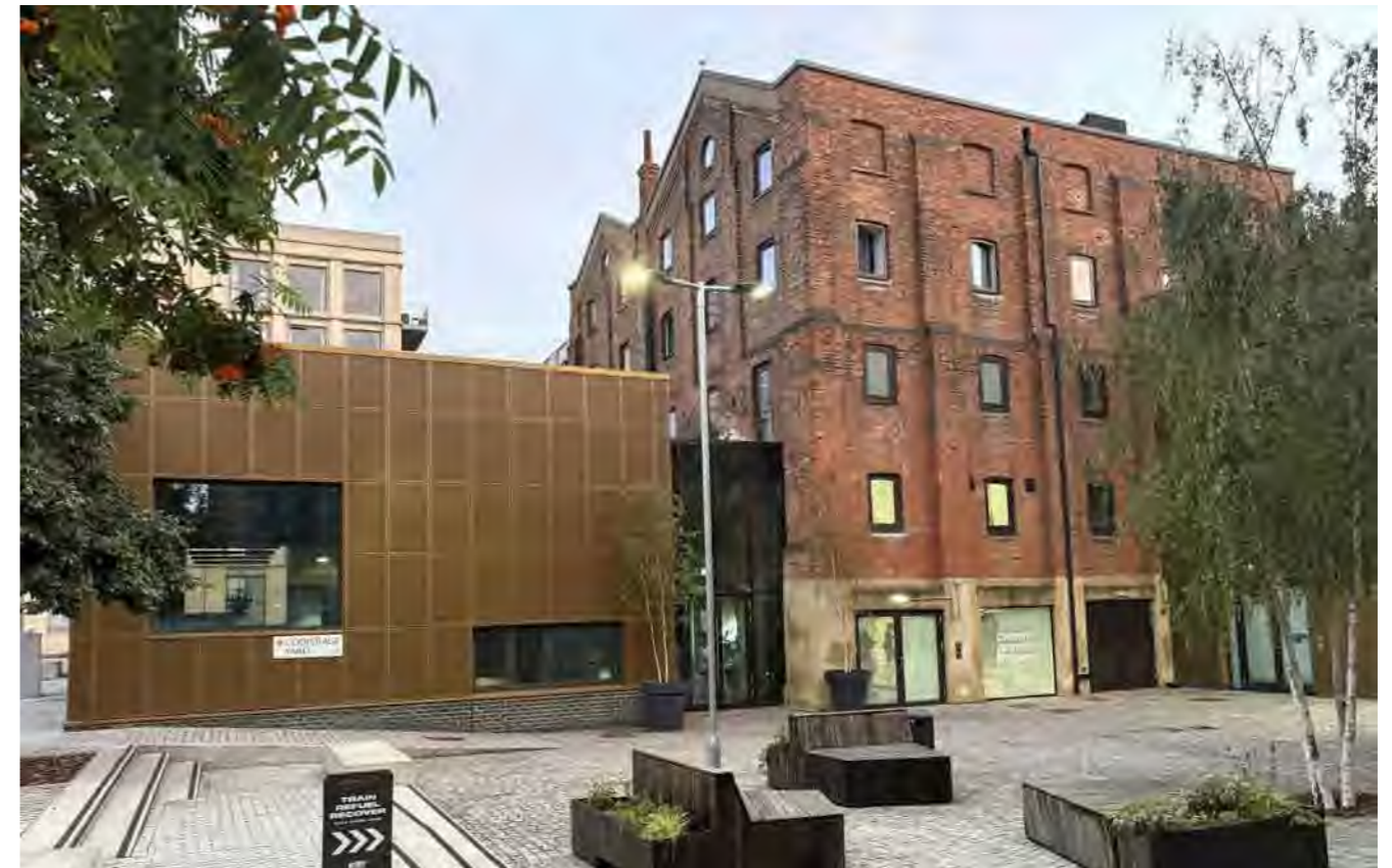
Fig 115 Retained warehouse building with contemporary extension accommodating community uses
