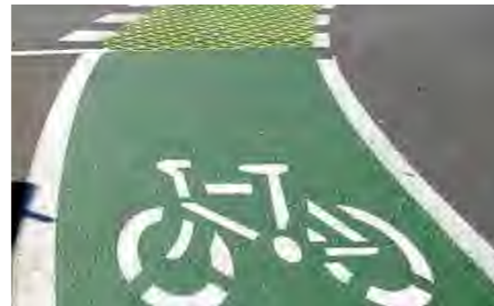
Fig 43 Top: Carriageway; asphalt Fig 44 Bottom: Cycleway; coloured asphalt
