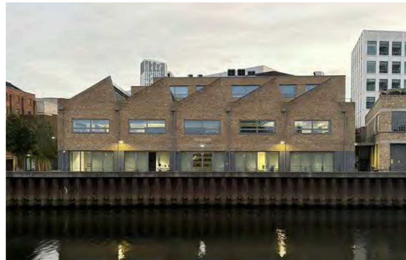
Fig 84 Saw-tooth roof to new brick building accommodating employment, responding to the area's rich industrial past.
