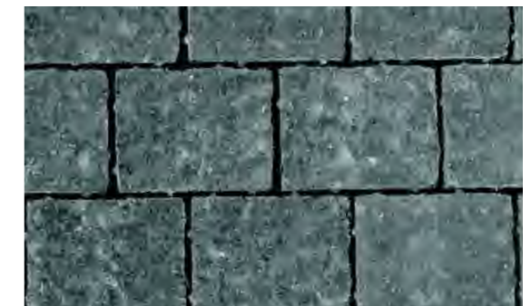
Fig 53 Top: Permeable linear paving Fig 54 Bottom: Permeable cobbles with built-in nibs to ensure sufficient joint width
