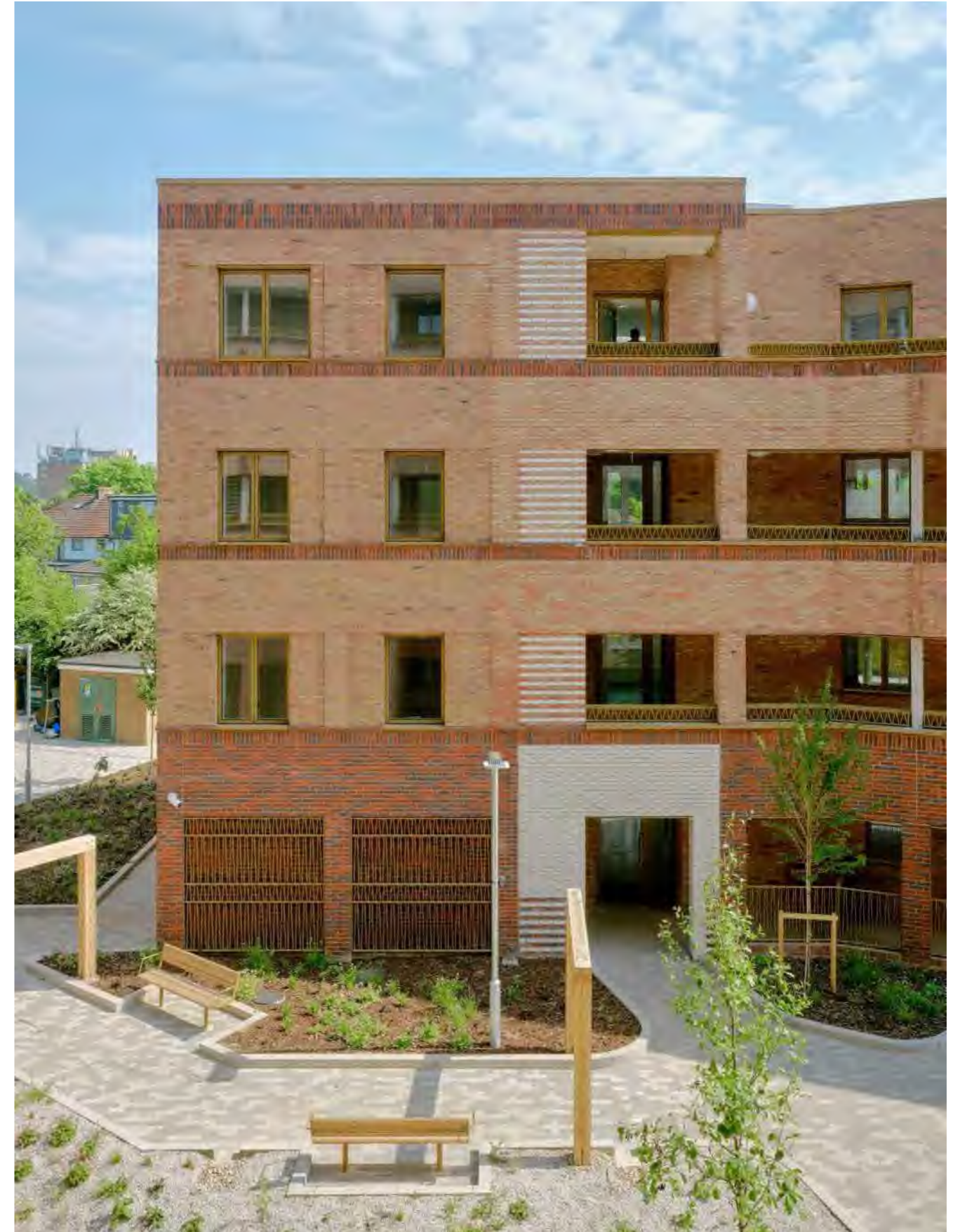
Fig 98 Low rise apartment building
